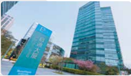
Siemen Electrical Apparatus Ltd. Suzhou, Shanghai Branch(APT Operating Company)
